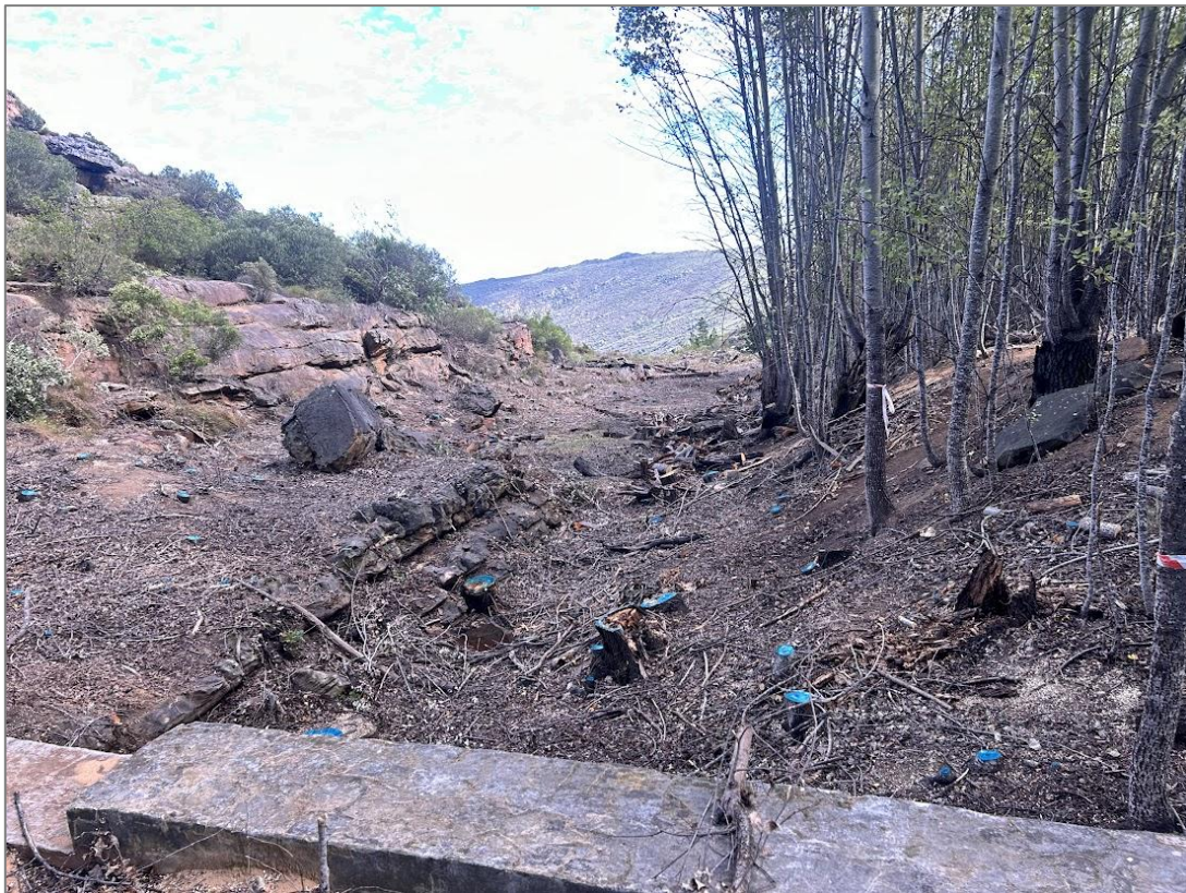
Photograph 21 Foothill stream downstream of Dam 5 (April 2026) – weir shown in foreground.
