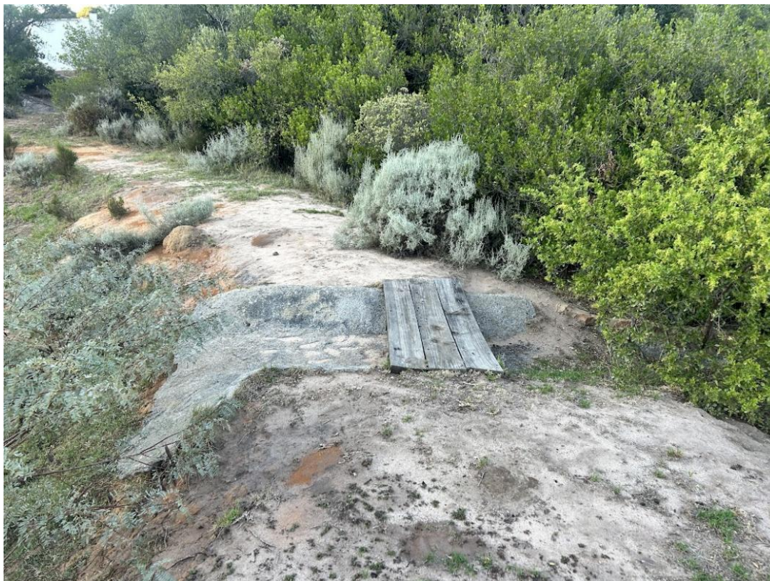
Photograph 16 Concrete spillway over the dam wall of Dam 4
