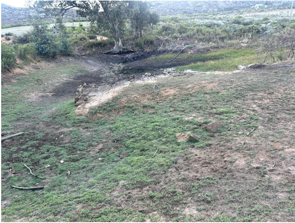
Photograph 18 Standing water in Dam 4 (April 2026)
