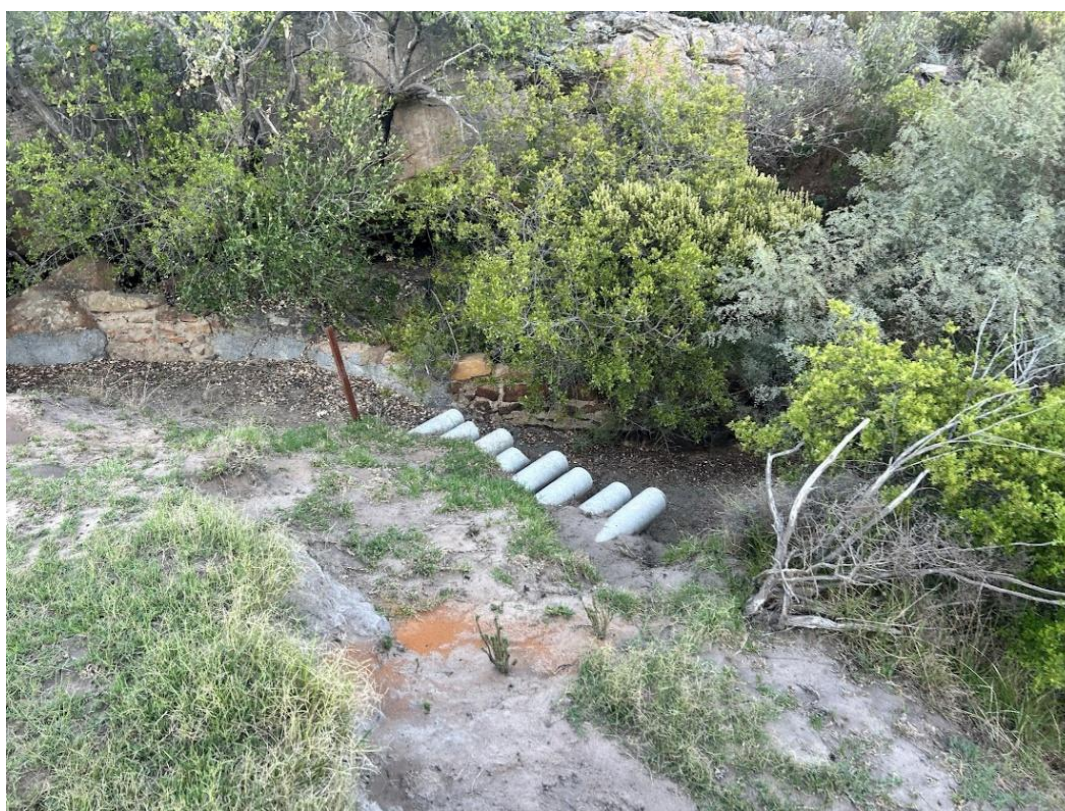
Photograph 17 Pipe outlets from Dam 4 into the concrete spillway
