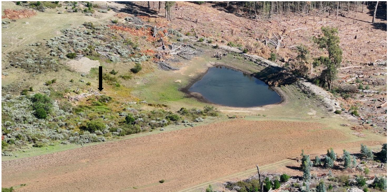
Photograph 2.5 Dam 1 viewed from the northeast
