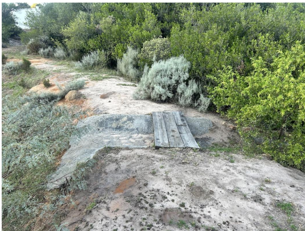
Photograph 2.13 Concrete spillway over the dam wall of Dam 4
