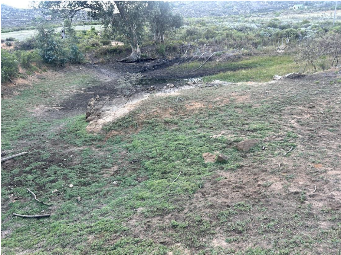
Photograph 2.15 Standing water in Dam 4 (April 2026)
