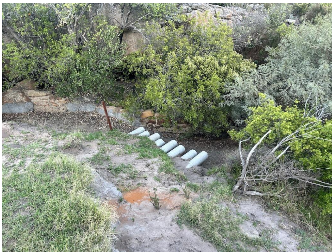
Photograph 2.14 Pipe outlets from Dam 4 into the concrete spillway
