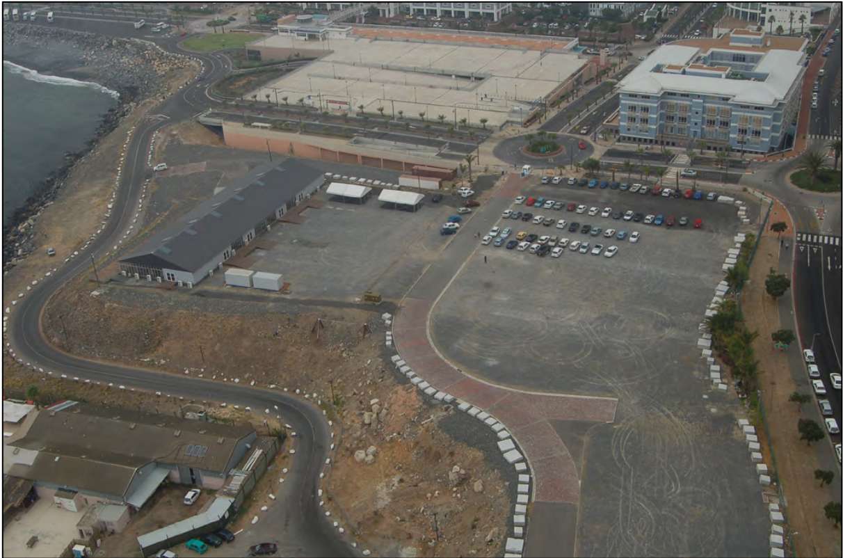
Plate 1: Aerial view looking east across a portion of the land reclamation project site showing the deep fill between Jetty Street and Beach Road on which the parking lot and black-roofed building are constructed (After: Baumann 2015).
